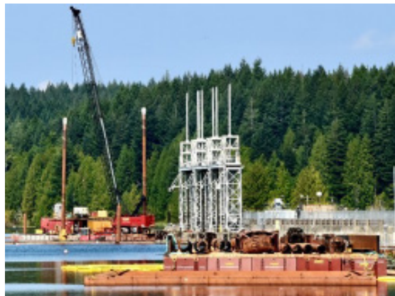
▶ John Hart Seismic Upgrade – Silt Curtain Installation
