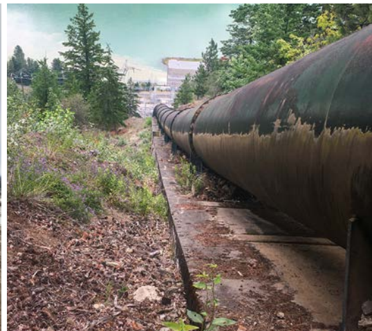
▶ Bridge River Strip & Recoat Penstock 1-4
