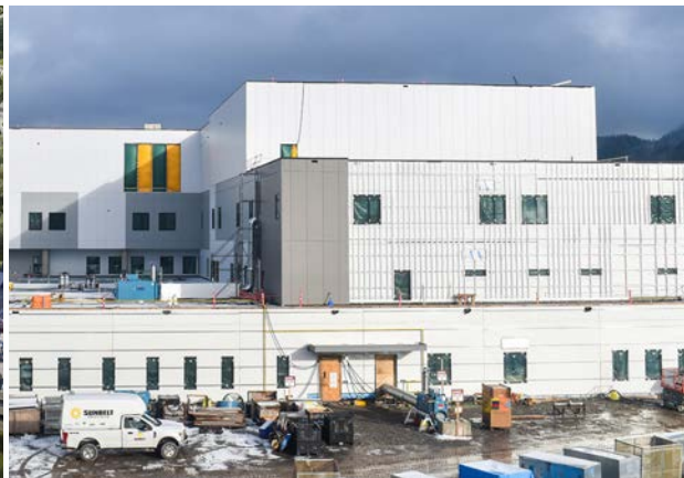
▶ Mills Memorial Hospital Construction
