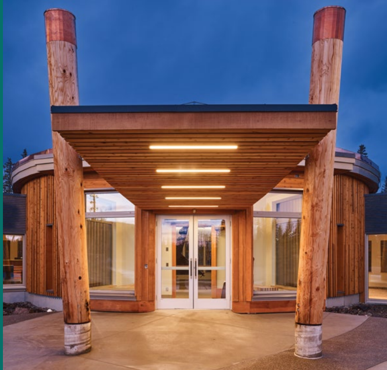
Nadleh Whut'enne Yah Administration and Cultural Building, Nadleh Whut'enne Yah Territory, Fort Fraser Architect: Evans Architecture & Joe Y Wai Architect | Photography: Martin Knowles
