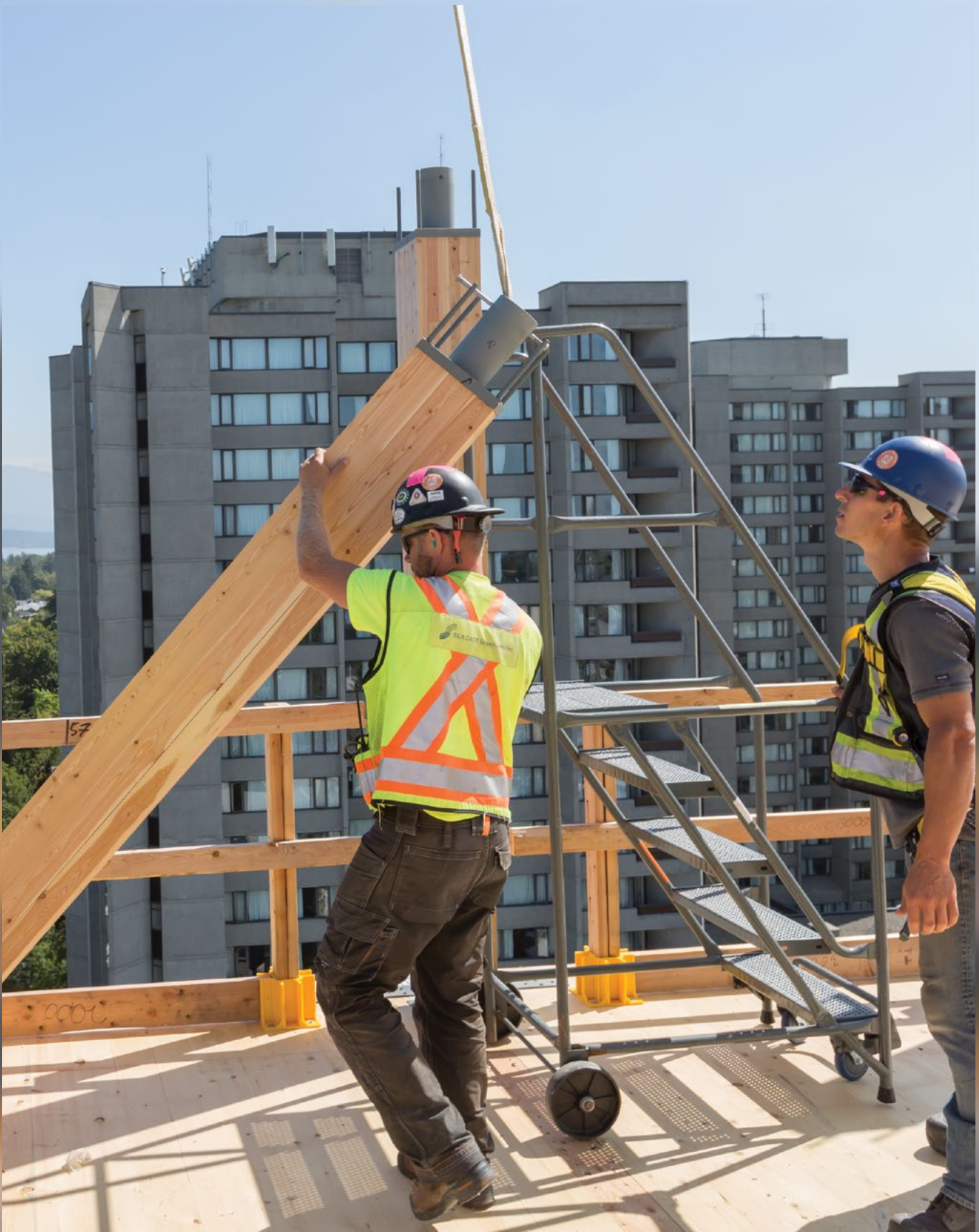
Installing mass timber at Tallwood House at Brock Commons, UBC, B.C.'s first tall mass timber building. Architect: Acton Ostry | Photography: Steven Errico
