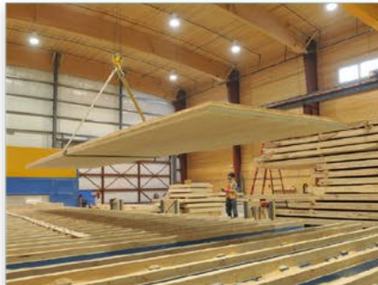
8 Structurlam mass timber facility, Penticton.
