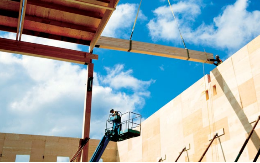
StructureCraft facility under construction in 2017, Abbotsford. Photo courtesy of StructureCraft Builders Inc
