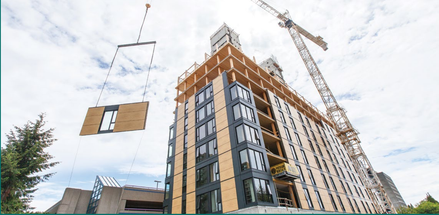
Construction of Brock Commons Tallwood House , University of British Columbia. At time of completion in 2017, the tallest mass timber building in the world. Architect: Acton Ostry | Photography: KK Law
